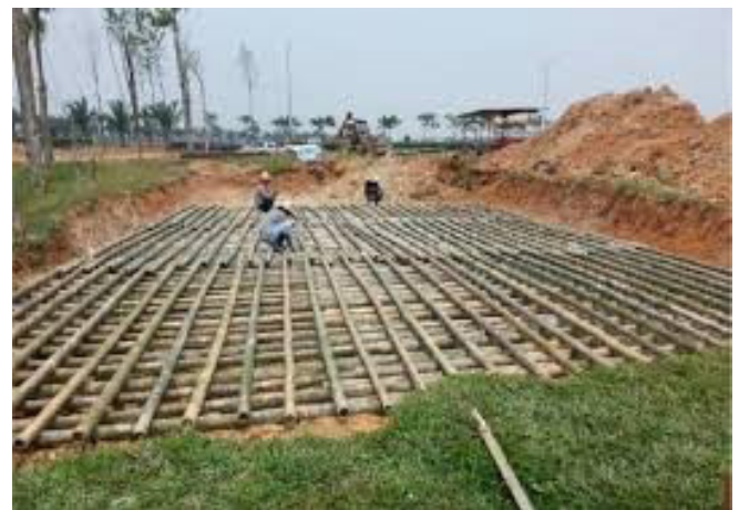
(a) Bamboo soil reinforcement (Gidon and Sahoo, 2020)
