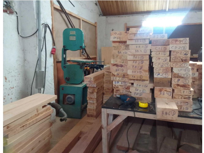
Ardhi Na Mbao workshop during pre-fabrication works for the upcoming Tiny Luxury Accommodation project
