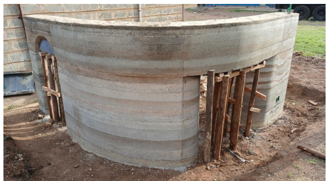
Rammed Earth Sample wall by Ardhi Na Mbao for the Maasai Mara Conservation Centre project.
