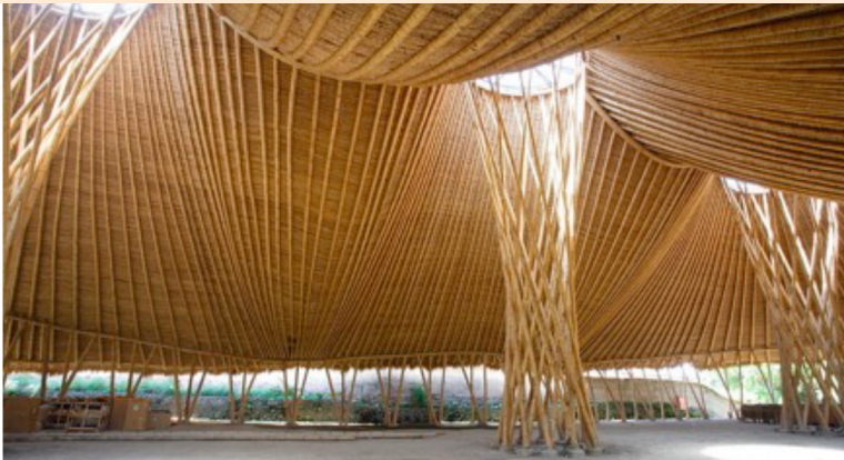
(a) Bamboo frame and roof (Krötsch, 2013)
