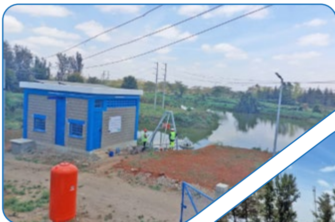
Intake works (3000m 3 /day) at Mbagathi River (EAPCC Dam)
