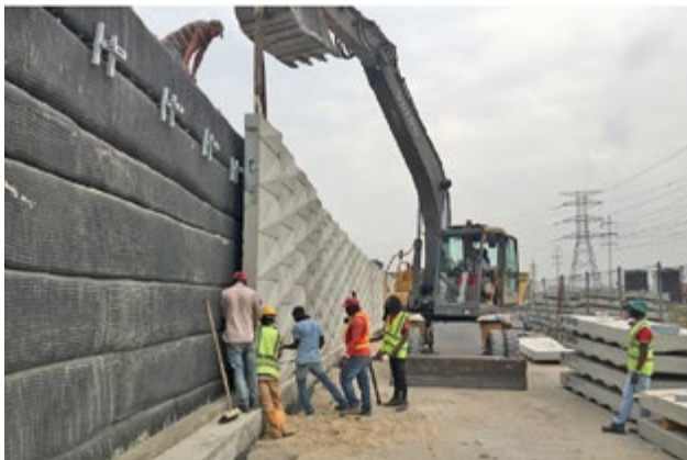
Figure 1: MSE structure with geogrid reinforcement, Lekki Expressway, Lagos, Nigeria
