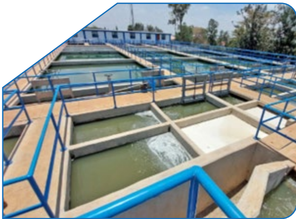
Flocculation basin and sedimentation tanks of the 12,000m 3 /day WTP
