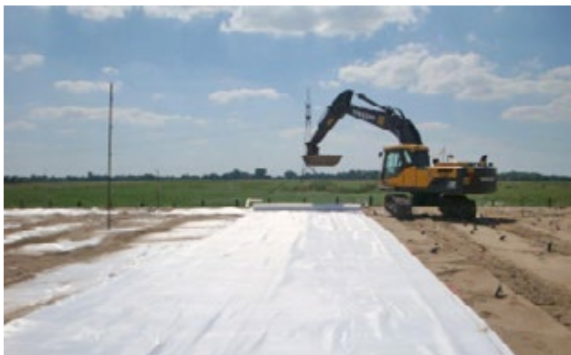
Figure 3: Basal reinforcement under embankment on soft sub-grade
