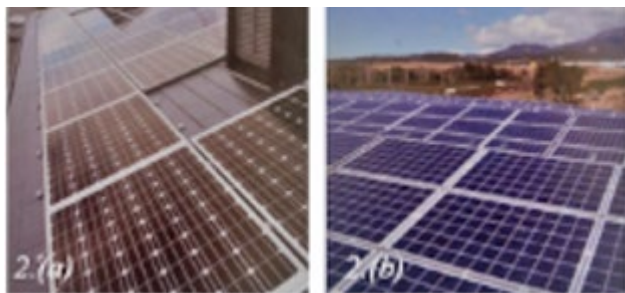
Fig. 2. (a) Show monocrystalline SW275 solar panels on a roof top system 16.225 kW installed at Hyogo Japan, while fig. 2. (b) Show SW250 polycrystalline panels in a 600kW solar power plant installed at Shizuoka Japan. Photos courtesy of Europe Solar Innovation Co., Ltd –Japan to which Europe Solar Innovation [EA] Co., Ltd-Kenya is affiliated.
