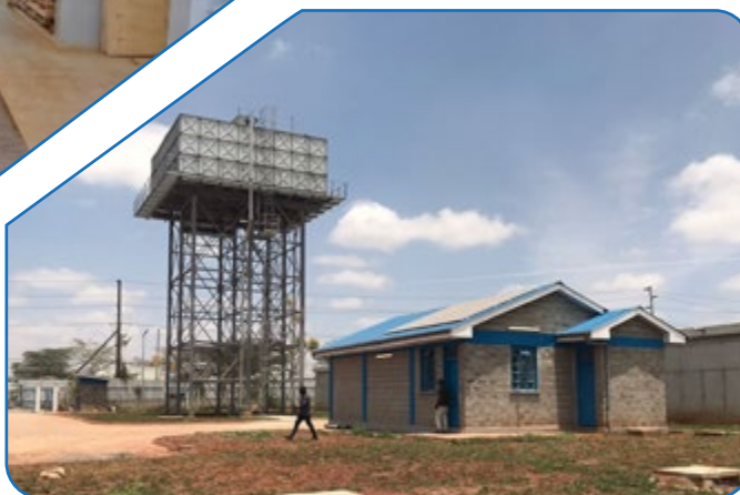
4500m 3 RC tank and 300m 3 Steel elevated tank at Syokimau. Pump House (2No 200m 3 /hr pumps)
