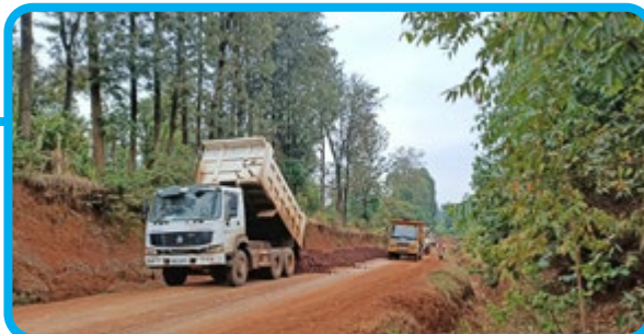
Gravel dumping at Imenti Central, Meru County.
