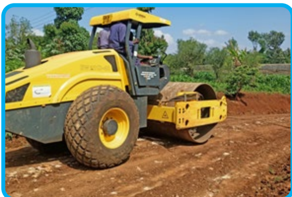
Road compaction works at Nakabune Nyaki East ward, Meru County.
