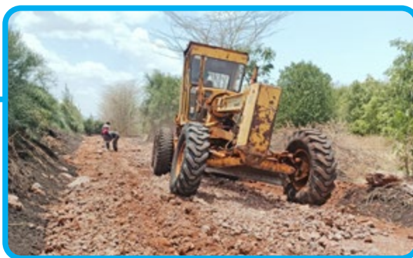
Gravel spreading at Kiirua Naari Ward, Meru County.
