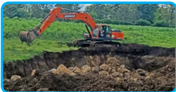
Overburden removal and gravel excavation in Nyaki East Ward, Meru County.
