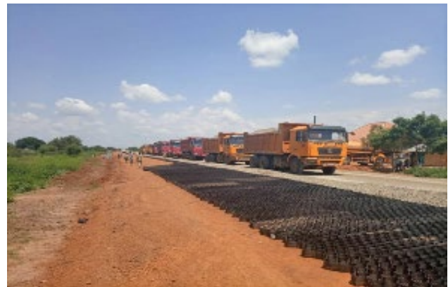
Figure 4: Neoloy geocells installed at Hoima Road, Uganda
