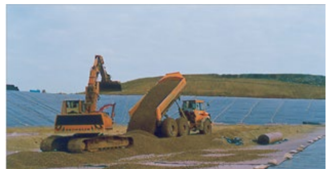
Figure 5: Nonwoven geotextile used as filtration/separation fabric
