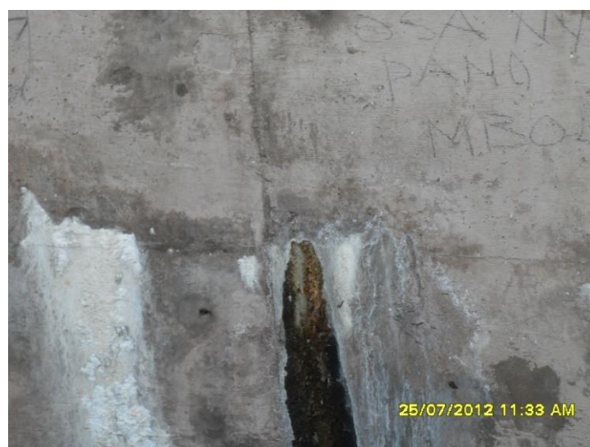
Figure 1. Efflorescence from a leaking water tank.
